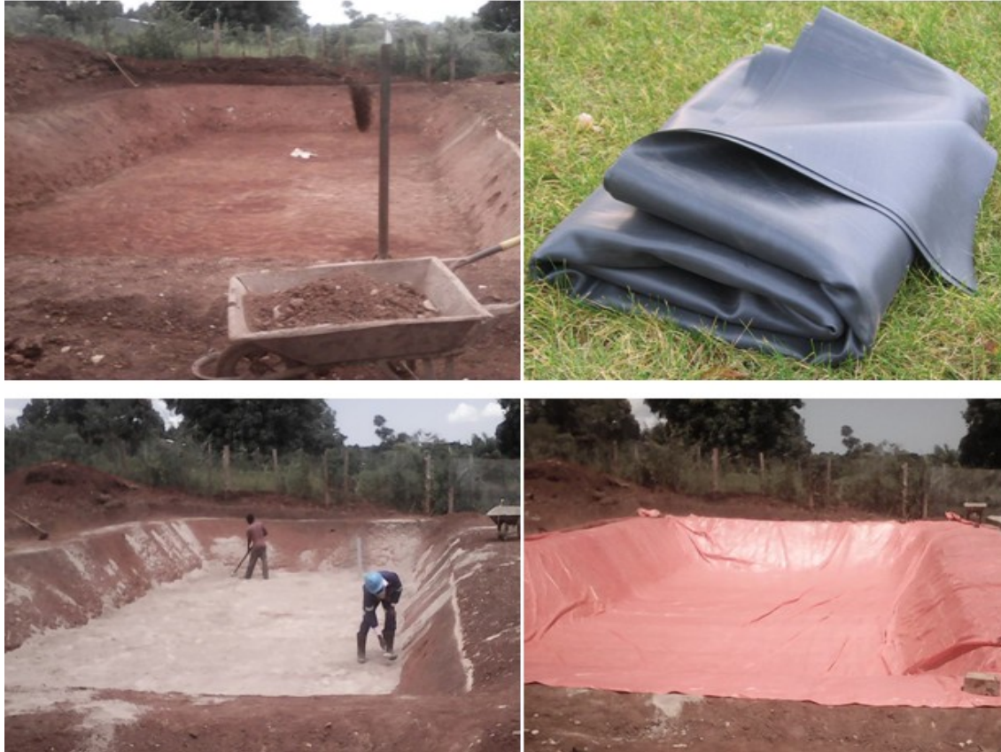
Figure 4.12 Runoff harvesting pond under construction in the study area
