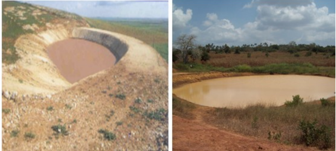
Figure 3.2 Excavated water Pans
